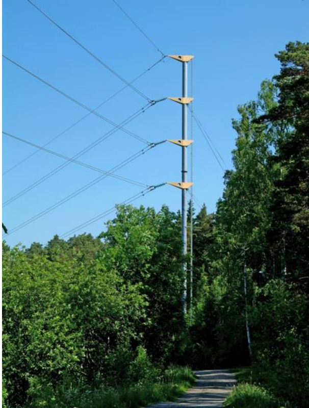
Figure 82 Examples of design towers, used to mitigate the visual effect of the transmission lines
