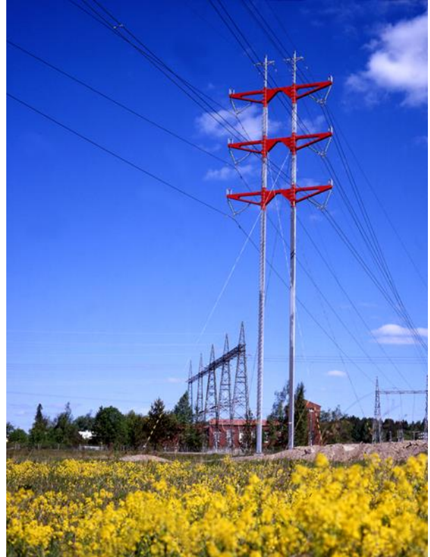
Figure 82 Examples of design towers, used to mitigate the visual effect of the transmission lines
