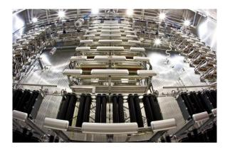
While converting AC electricity to DC (and vice versa) the valves pictured above switch 1,650 times per second and are controlled via fibre optic cables.
